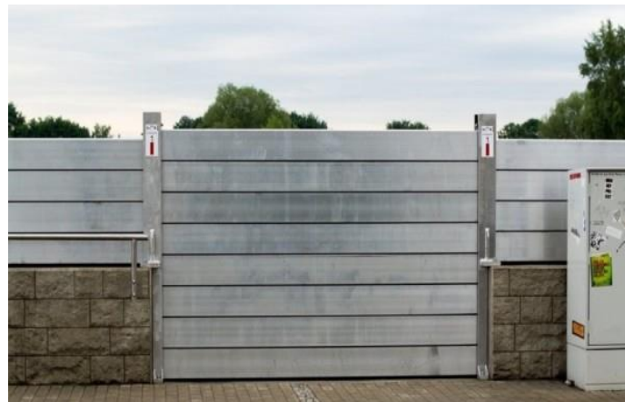
Figure 4. Pre-assembled metal panels
